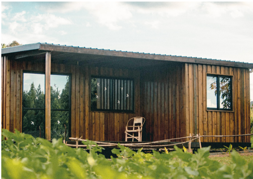
One of Easy Housing's modular timber homes. Picture credit: Easy Housing
