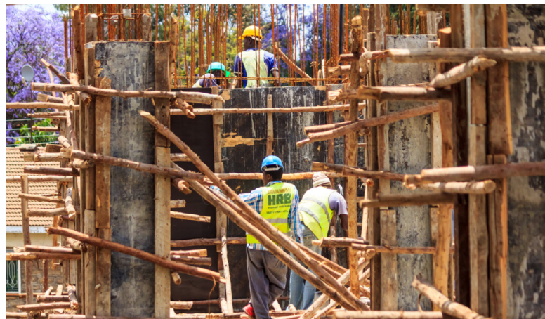
Construction work in Nairobi. Picture credit: Joshua Wanyama
