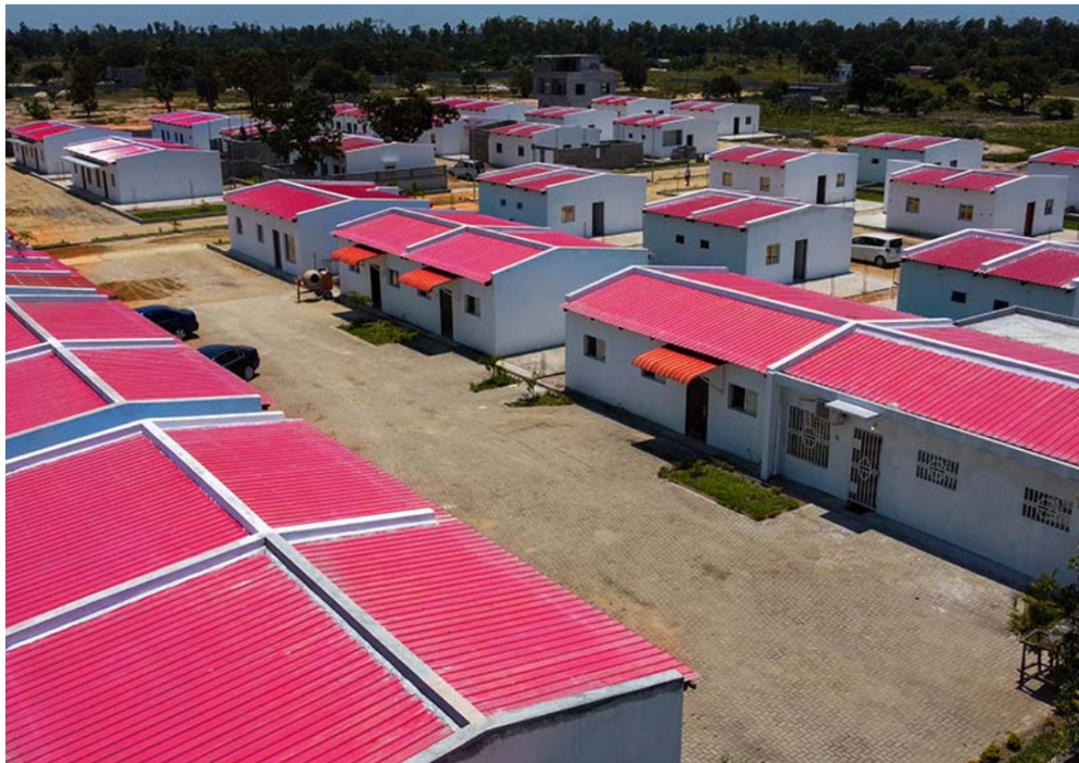
Casa Real's development in Beira. Picture credit: Casa Real
