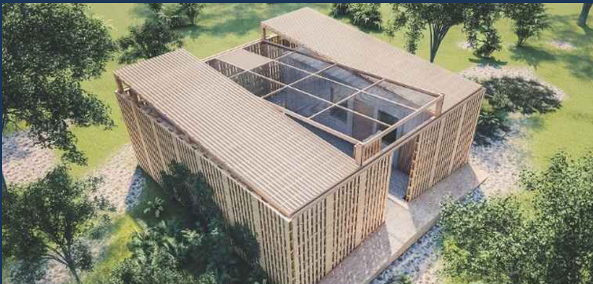
The Mahali Hub is an innovative, modular 'house in a box' which won the City of Cape Town's My Clean Green Home competition in 2021. It's designed as a net-zero concept home which incorporates many of the principles we have mentioned above: solar power generation, energy efficient appliances, passive cooling, rainwater harvesting and autonomous food production. Picture credit: Team Mahali.
